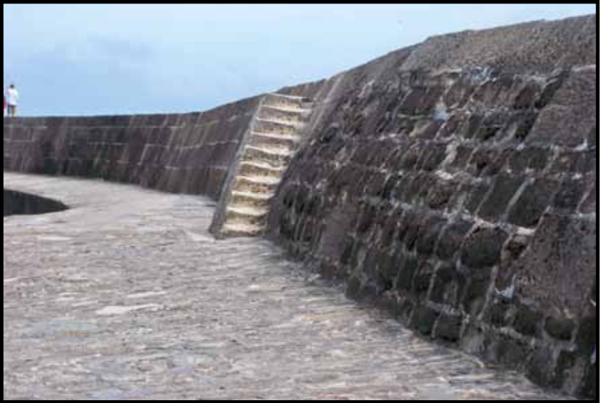
Steps on the southern arm. Though Granny's Teeth (see photo below) are often assumed to be the site of Louisa Musgrove's fall in Persuasion, the age, location, and condition of these steps further along the wall make them more likely the flight Austen described.
